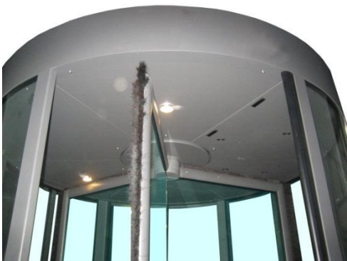
SINGLE-PRESENCE DETECTION SENSORS WITHIN A REVOLVING DOOR'S SECTOR
